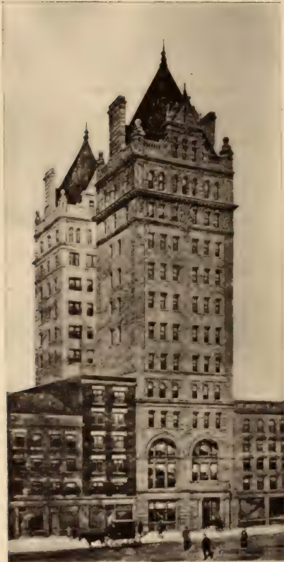
LAWYERS' TITLE INSURANCE CO.'S BUILDING. Maiden Lane Front. Chas. C. Haight, Architect.
